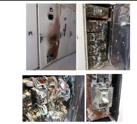
Fire at the Main Power Distribution Panel at a bottling industry; fortunately, the Company had the main Panel Room at a separate area away from the main manufacturing facility.
